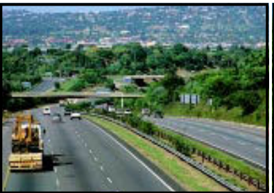
Transportation: Freeway, Pretoria
